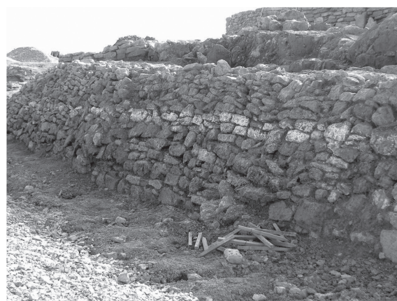
Figure 12. White line on the internal scarpment of the moat (N side) corresponding to \text{CaCO}_3 precipitation. The thickness of the white line is about 20 cm.
